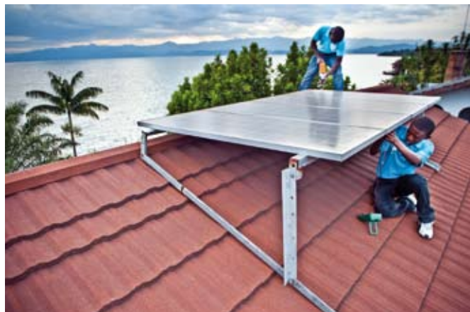
Energise Africa: BBOX technicians fix solar panels to a roof in the Democratic Republic of Congo.
